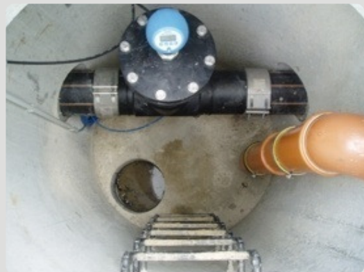
Top view on measurement point in manhole
